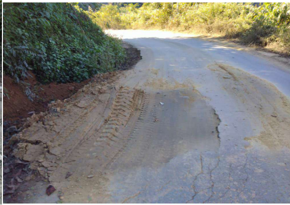
Photo of Pot holes between ch: 69/00 kmp to 110/00 kmp on NH-6
