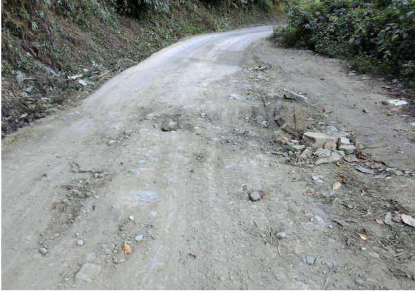
Photo of Pot holes between ch: 69/00 kmp to 110/00 kmp on NH-6
